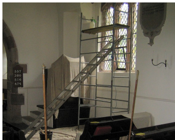
Llanvapley Church running repairs – God bless this mess!
